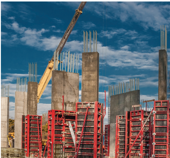
Columns and beams
