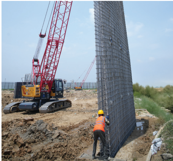
Diaphragm Wall/Retaining wall
